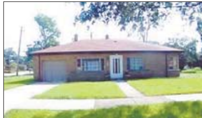
845 CATHERINE, LA GRANGE PARK —$349,900. Great investment opportunity on oversized lot. Teardown property in sought-after Harding Woods area, across from new construction and forest preserve.
